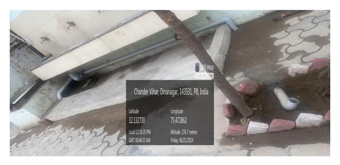
Waste water from A.C. Pipe is collected for use in batteries and chemistry labs.
